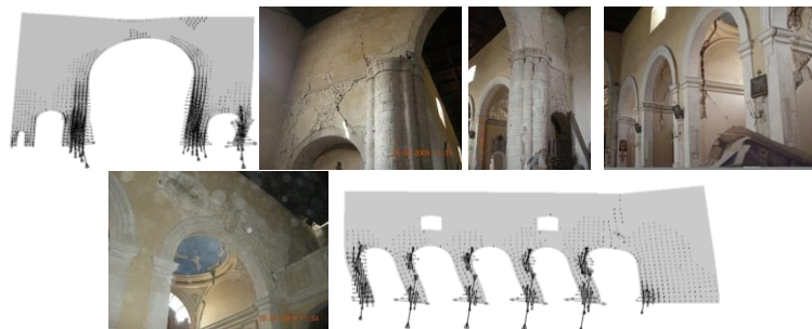
Figure 9 SG - seismic damage and analysis results: triumphal arch (T7) and arcade (L3).
