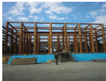
Fig. 3: Timber frame erection.
