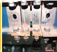
Bottom flange fracture
